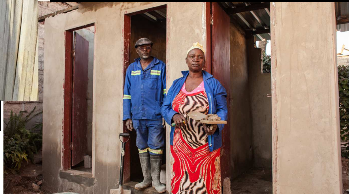
Communities provide skilled and unskill labour including women to construct Improved Public Sanitation Facilities at Masala Market, Ndola, Zambia
