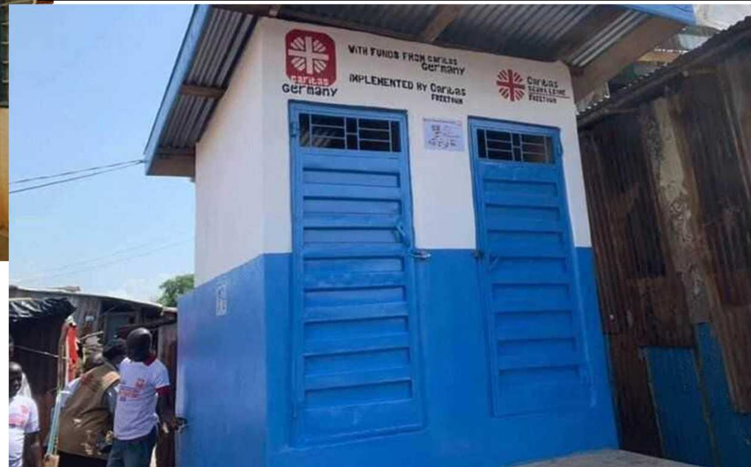
Ventilated Improved Pit (VIP) Latrine, Colbot, Freetown, Sierra Leone
